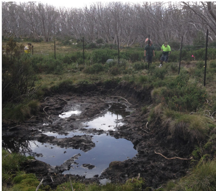
Exclusion fencing being erected at Mount Bullfight
