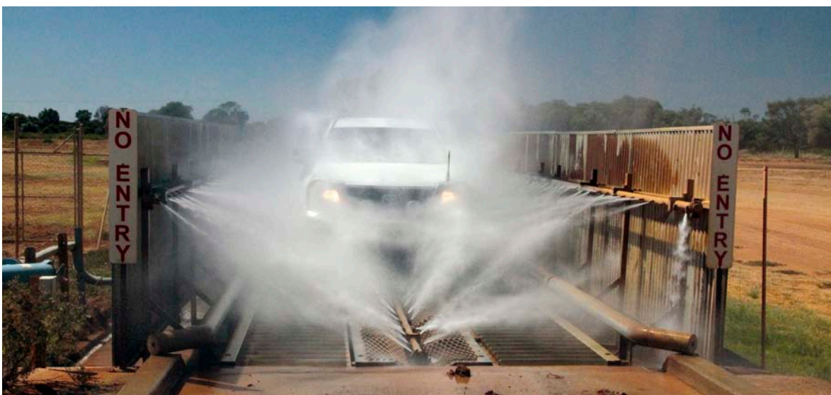
Clean-down facilities. (a) A gamba grass clean-down and inspection bay near Cooktown in Far North Queensland. Coarse aggregate is the base of the bay where physical inspections are carried out, before the vehicle is cleaned using high-pressure water pumped from tanks. (b) A local government high-pressure clean-down facility in operation in Queensland.
